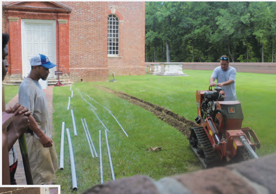
Above: Chris Hanley and his team from Hanley Electrical Services, LLC of White Stone use a ditch witch to trench conduits under the churchyard wall and several brick pathways from the church to the Chase Center, where they will provide communication lines for the moisture monitoring system and church security upgrade. Anna Rhodes, senior archaeologist with the Fairfield Foundation and Data Investigations, mapped the conduit routes to document their precise locations following guidelines from the Virginia Department of Historic Resources, which has easement oversight on everything inside the churchyard wall.
