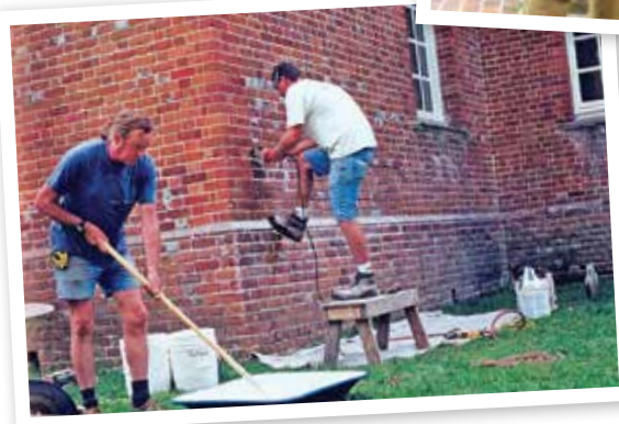
Tidewater Preservation conservators Greg Cowan (left) prepares mortar while Chris Anderson removes decayed mortar joints during repointing work in 2000.
